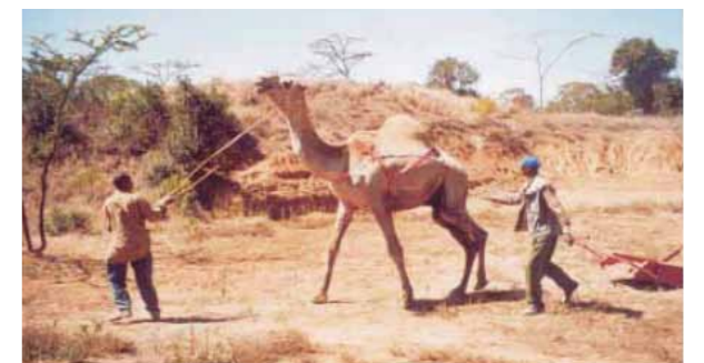
Camel de silting a dam (Source: Chris Field)
