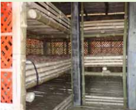
Figure 1: A potato storage ambient store constructed with local materials
